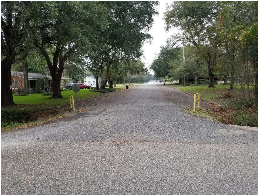
6. Intersection of South Street and Purdy Ave looking north along Purdy Ave.
