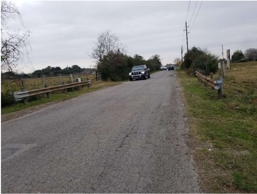
25. Looking north along FM 1489 near drainage channel.
