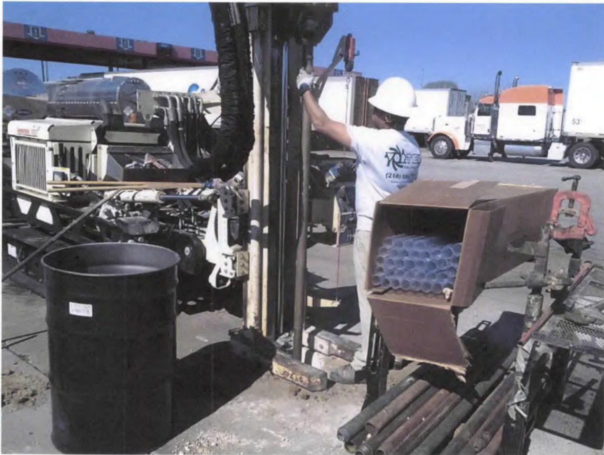
Geoprobe drilling rig used to advance borehole
