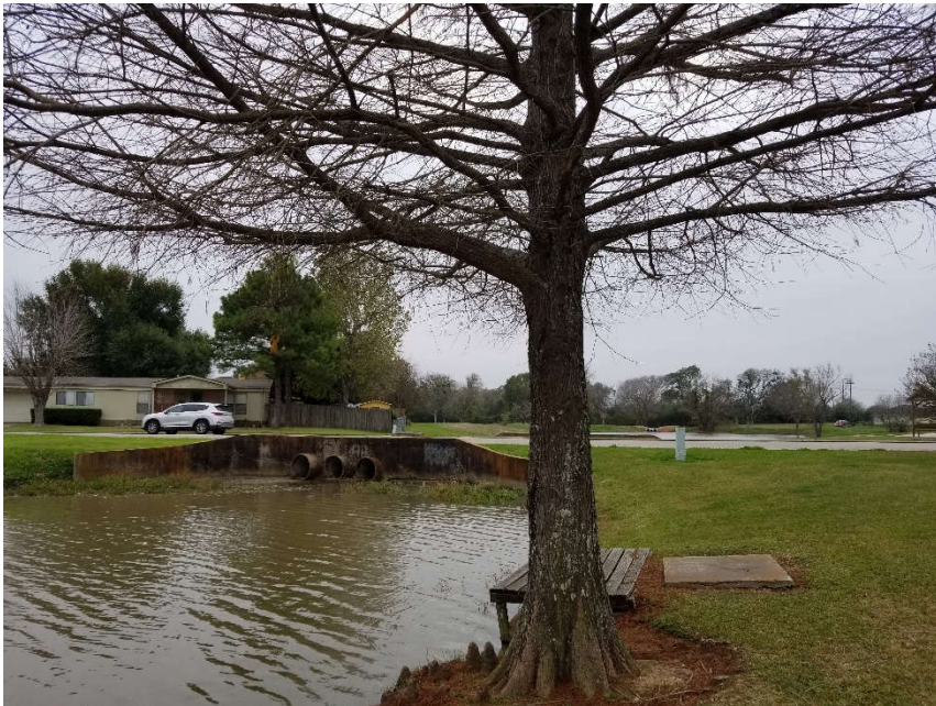
18. Concrete culvert along Lakeside Drive.
