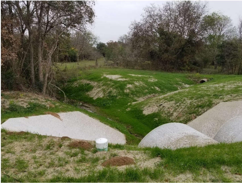
17. Ditch perpendicular to Lakeside Drive. Looking northwest.
