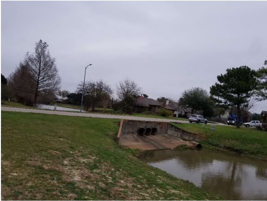
19. Concrete culvert along Lakeside Drive.
