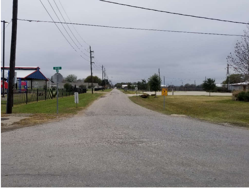
1. From Baines Street looking west along 5 th Street.
