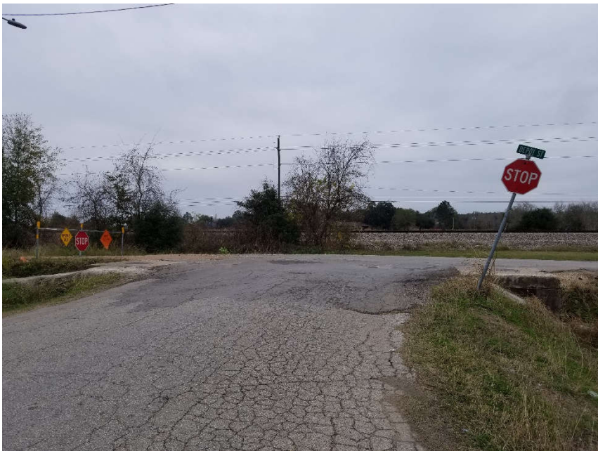
28. Intersection of Depot Street and Stalknecht Road looking south.
