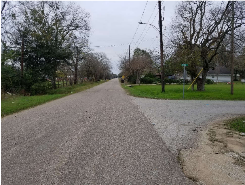
27. Intersection of 1 st Street and Rouse Ave, looking east along 1 st Street.
