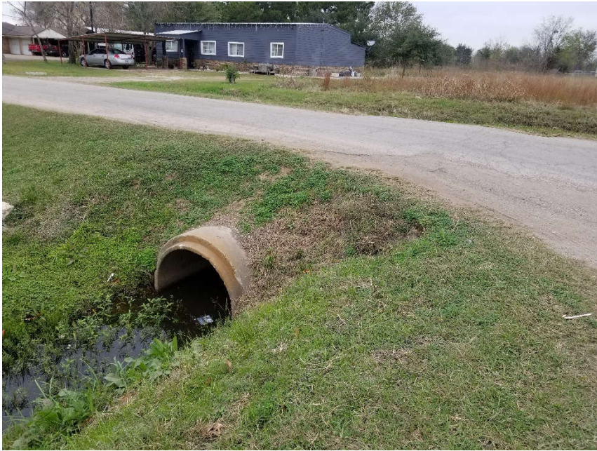
23. Gassner Road at Drainage Channel.
