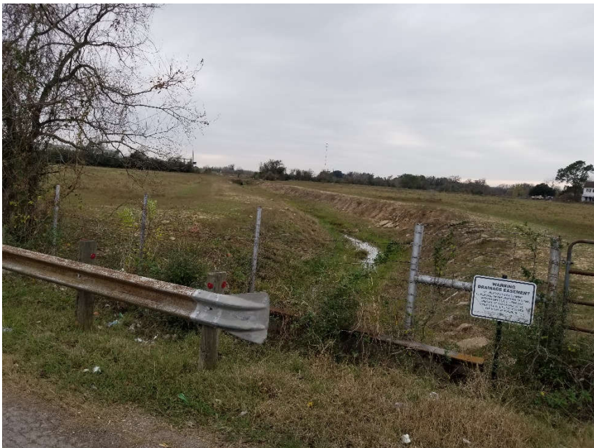
22. Gassner Road at Bacon Street (drain).
