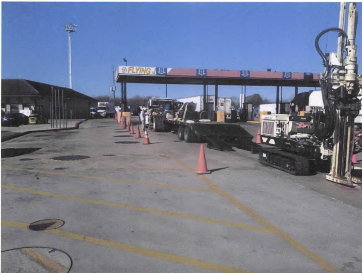
Facing west, showing location of borehole north of USTs.
